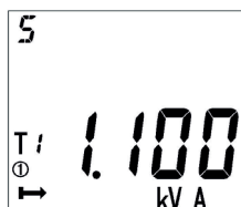
Current total apparent power 1.100kVA
