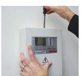
**10.** Secure the two fixing screws top and bottom.
