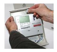
**6.** Remove the three plastic plugs to reveal the fixing points of the base.
